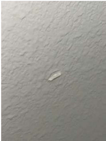
Front Entry closet
