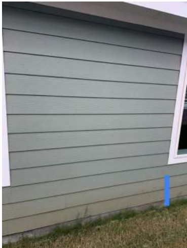
Side Yard Exterior Walls
