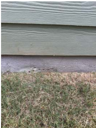
Right Side Yard
