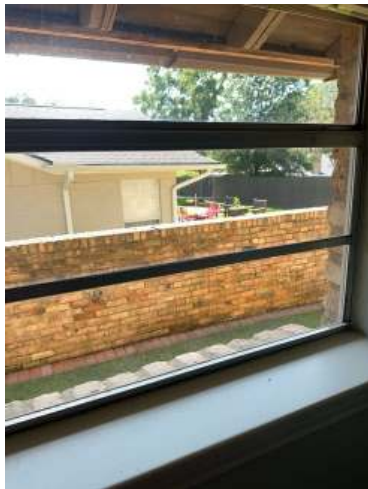
Perspective of single hung windows throughout the home. Bedroom 2
