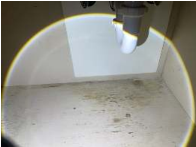
Fungal growth was observed at the back of the sink cabinet. We recommend having a qualified professional evaluate and address this issue. Bathroom, Hallway
