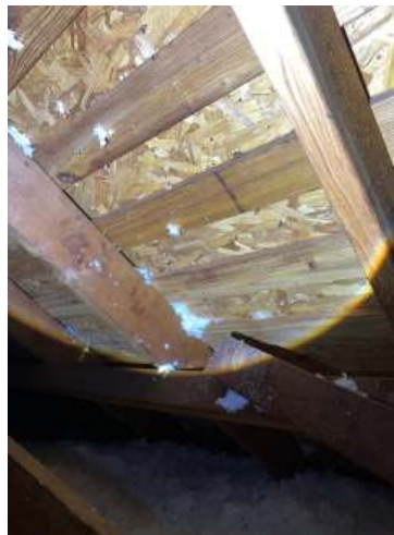
View of attic structure.
