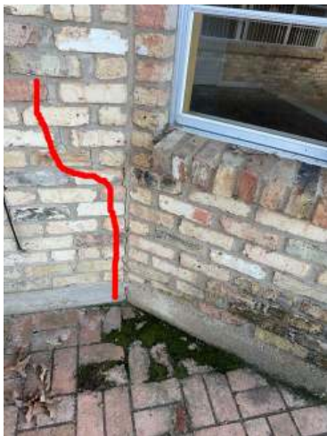
Rear, Back Yard, Exterior Walls
