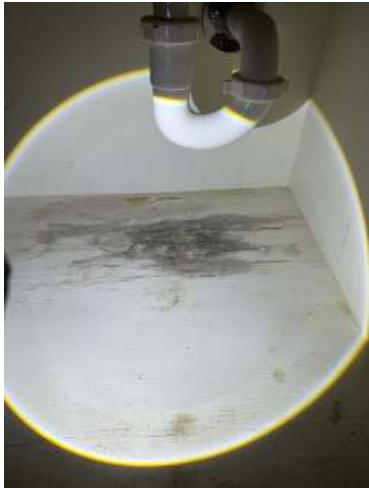
Fungal growth was observed at the back of the sink cabinet. We recommend having a qualified professional evaluate and address this issue. Bathroom, Hallway
