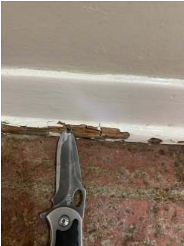
Knife point easily enters the wood trim piece.
