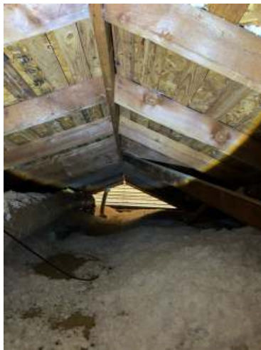
View of attic structure and gable vent opening to the front yard.
