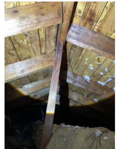
View of attic structure.
