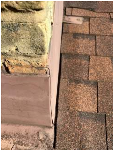
Caulking upgrade on the flashing around the fireplace chimney. Roof
