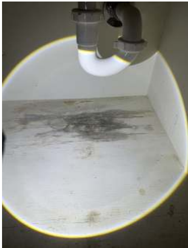
Biological fungal growth in base of cabinet. Hallway Bathroom
