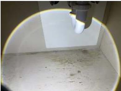
Biological fungal growth in base of cabinet. Hallway Bathroom
