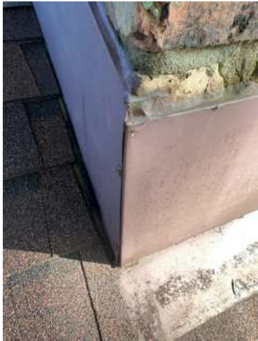
Caulking upgrade on the flashing around the fireplace chimney.
